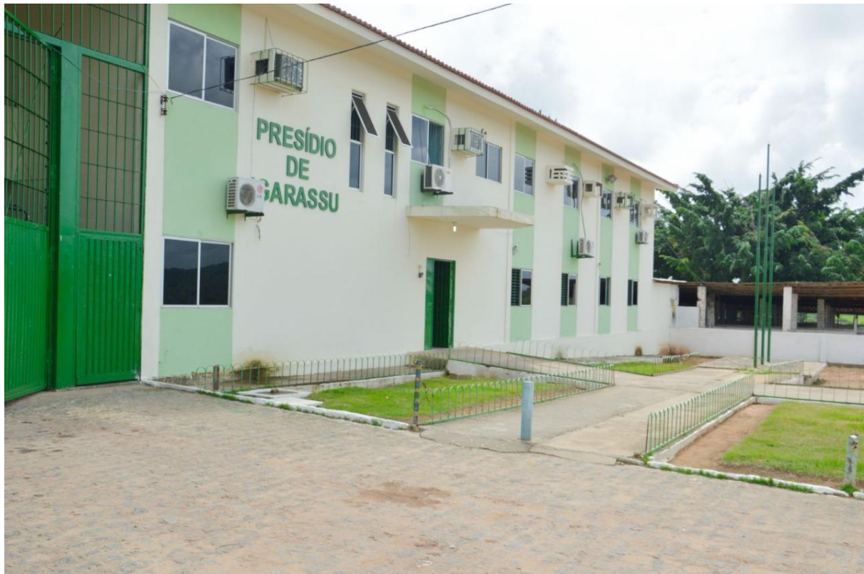
Igarassu Correctional Facility, Pernambuco (PE)
